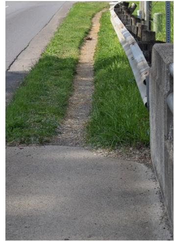
Sidewalk gap along 21st Street has led to this desire path
