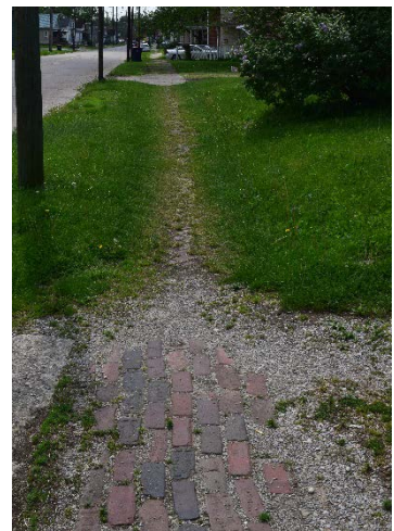
Sidewalk gap along National Drive caused this desire path
