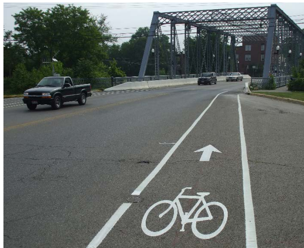
Eastbound bike lane on East Main Street
